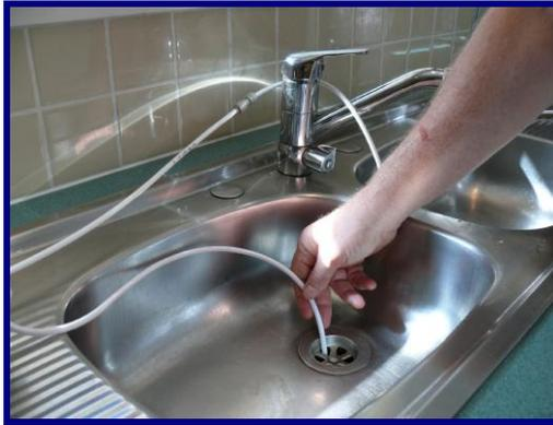
4. Reverse Osmosis Systems produces waste water, so place the drain line directly down the kitchen sink to dispose of this waste water
