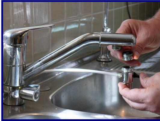
1. **Screw off the strainer from the kitchen tap, then connect the diverter valve to kitchen mixer tap (using the adaptor provided if required)**
